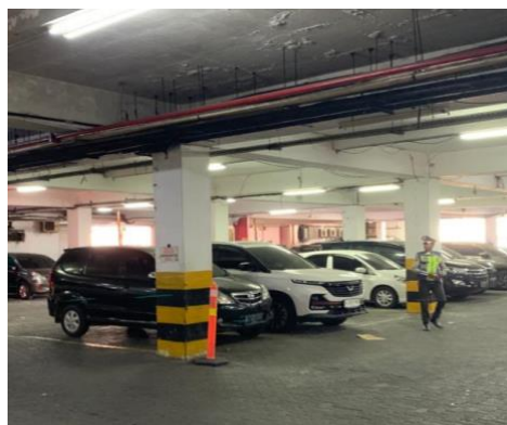
Gambar 2 Parkiran mobil di basement .
